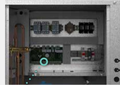
Rheem Commercial Heat Pumps (Split System) can be connected to a customer's Building Management System (BMS) or Building Automation System (BAS) via an interface card. Modbus or BACnet interface cards are available as accessories.
