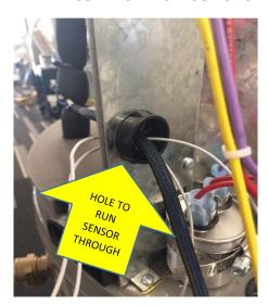
THIS IS WHERE THE CONDENSATE SENSOR IS STRUNG TO PLACE INTO THE PAN
